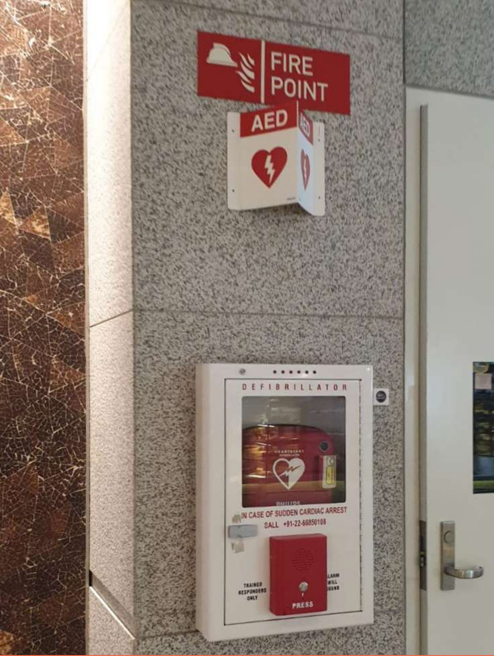
Image 6.1 Emergency Infrastructure Photo Credits: Dr. Gaurav Raheja
