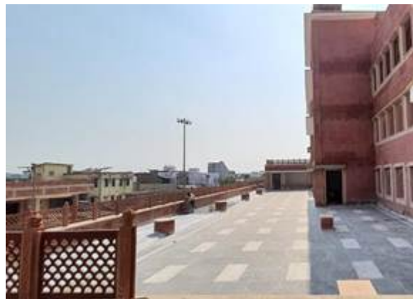
Open air Cafeteria at first floor
