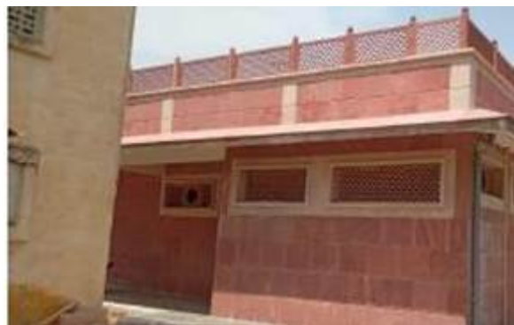
Toilet Block – Bus Stand
